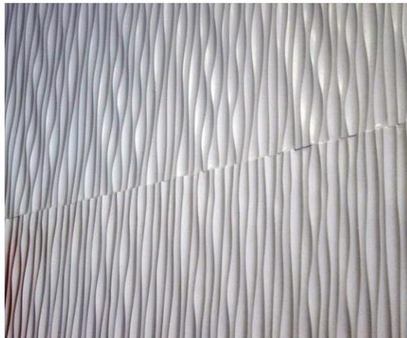
**PICTURE SAMPLE OF IMPROPERLY INSTALLED PATTERN**
