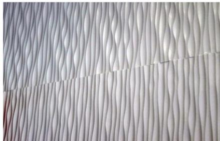
**PICTURE SAMPLE OF IMPROPERLY INSTALLED PATTERN**
